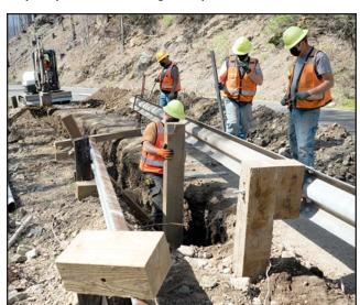
The other part of the Bridge Crew was busy replacing guardrails along Blue River Road, leading to the Blue River Dam. Existing guardrails there were fire-damaged as well as hit by falling trees. Drivers will notice the new guardrails are higher and closer to the road than the previous decades-old guardrail to meet current safety standards.
