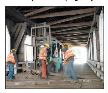
Lane County's Bridge Crew wa busy last week replacing about 80 damaged deck boards throughout the Goodpasture Covered Bridge. Increased traffic there had caused accelerated wear and tear. THe work was done to help protect the stringers underneath (which support the bridge deck) and help keep the structure in good repair.
