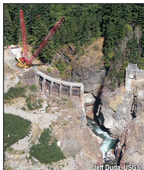
Glines Canyon dam removal on September 3, 2014.
