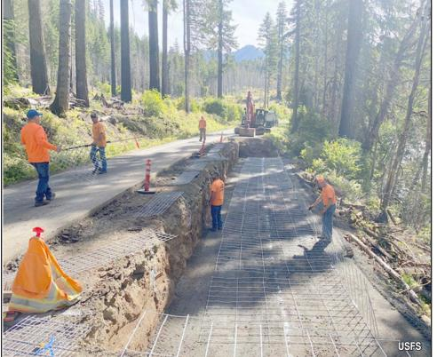
Reconstruction work on sections of USFS Road 19 (Aufderheide Drive) included welded-wire wall construction to address a failing road fill. Activities that were underway this summer will resume in 2024.
