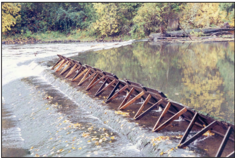
Lake Oswego Public Library The diversion dam as it appears today at relatively low river levels. All that remains is the concrete foundation, although some remnants of the structure can still be seen on the far shore.
