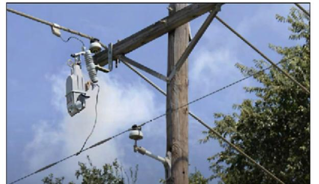
During an interruption of service, existing expulsion fuses on powerlines vent exhaust gases.
