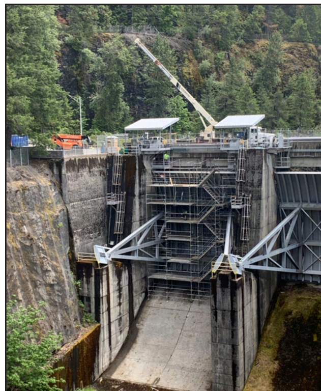
Workers erected scaffolding while painting the spillway gate 1 at Cougar Dam.
